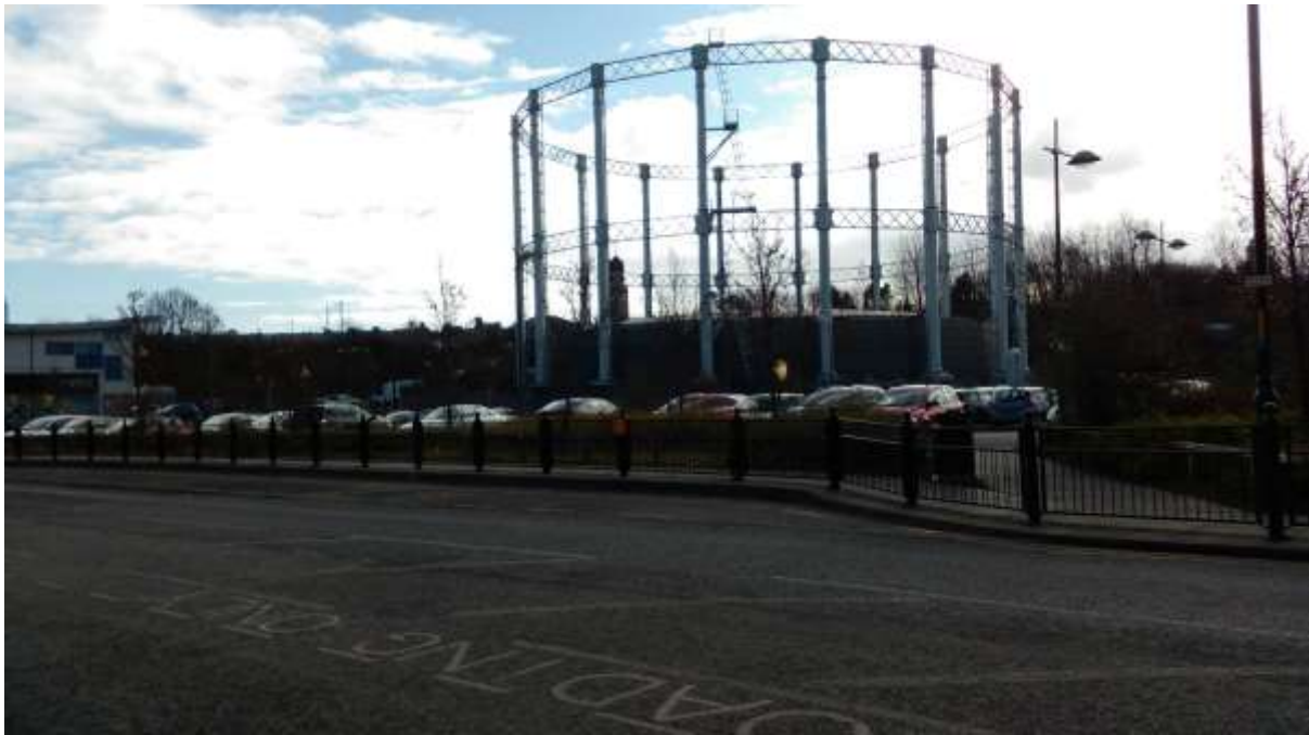
PLATE 1: THE GARDEN LANE-OYSTON STREET CAR PARK AND GAS RING.
